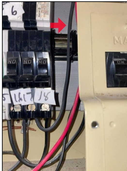
Wire crossing bus connections
