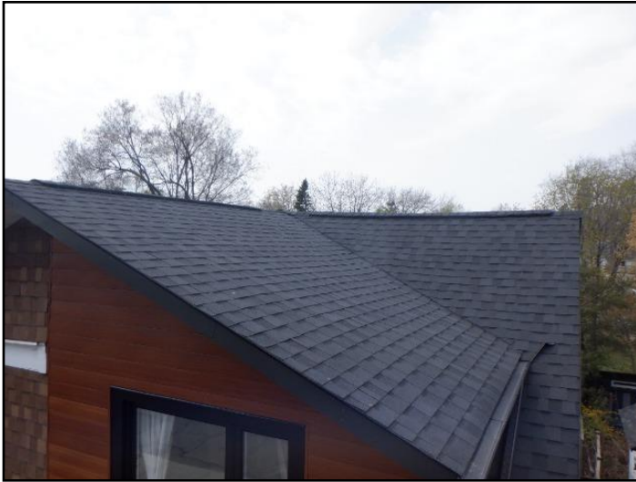
Asphalt shingles
