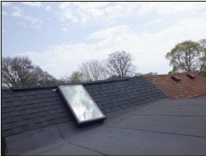
Modified bitumen membrane
