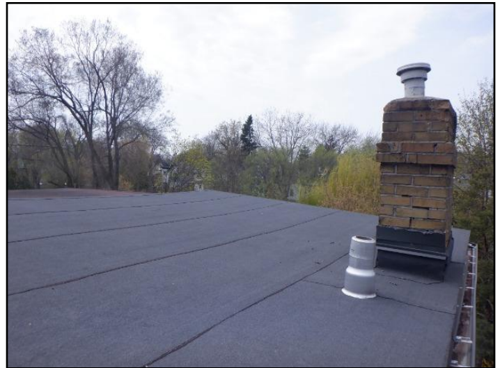
Modified bitumen membrane
