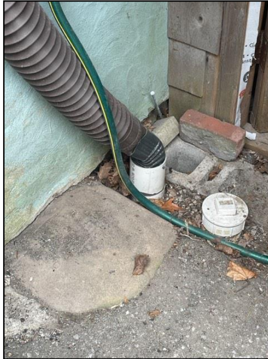
Downspouts that discharge below grade may...
