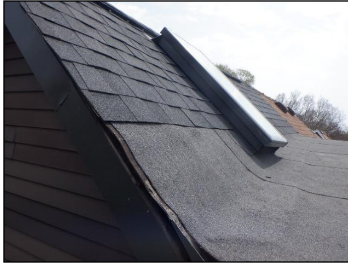
Skylight(s) - vulnerable area for leaks
