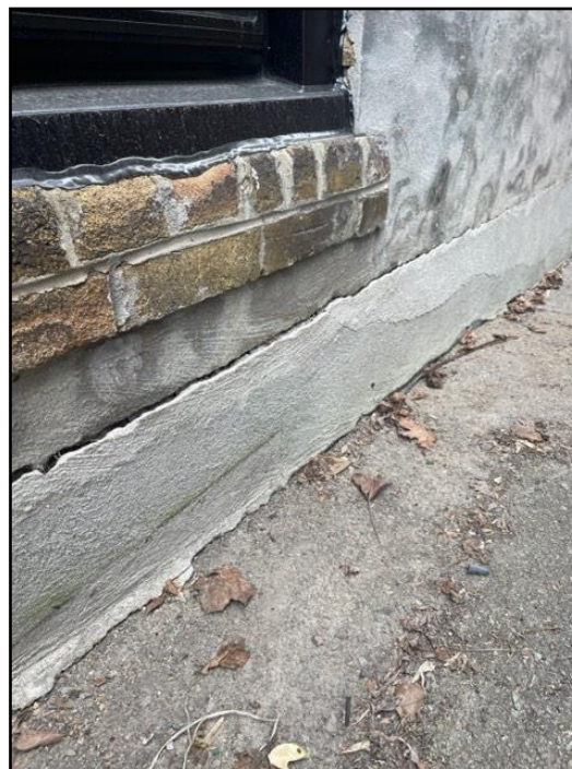
Parging damaged
